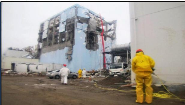
**Figure 12:** Fukushima's Unit 4 after a hydrogen explosion rips apart the 3<sup>rd</sup>, 4<sup>th</sup>, and 5<sup>th</sup> floor. Photo courtesy of Forbes: <http://www.forbes.com/sites/williampentland/2013/12/30/yakuza-gangsters-recruit-homeless-men-for-fukushima-nuclear-clean-up/>
