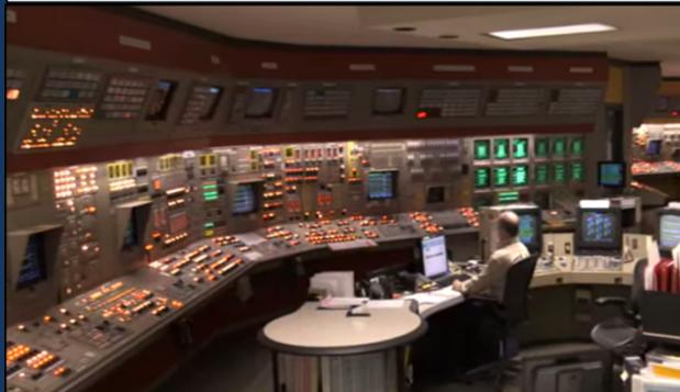
**Figure 3:** Darlington Nuclear Power Plant. Control room featuring multiple consuls where data fed from SCADA systems is relayed to control room workers. Note that many of these systems failed during the long power duration issues faced at Fukushima. The 2003 Northeast Blackout did not see widespread control room issues, however one automated process failed to perform from SCADA based controls in the Fermi 2 nuclear plant in Toledo, OH. It took 26 hours to resolve the issue.
